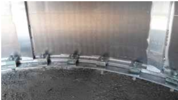
Silo Fixing Footings
